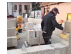
Hempcrete block construction
