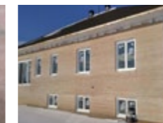
Building with hempcrete
