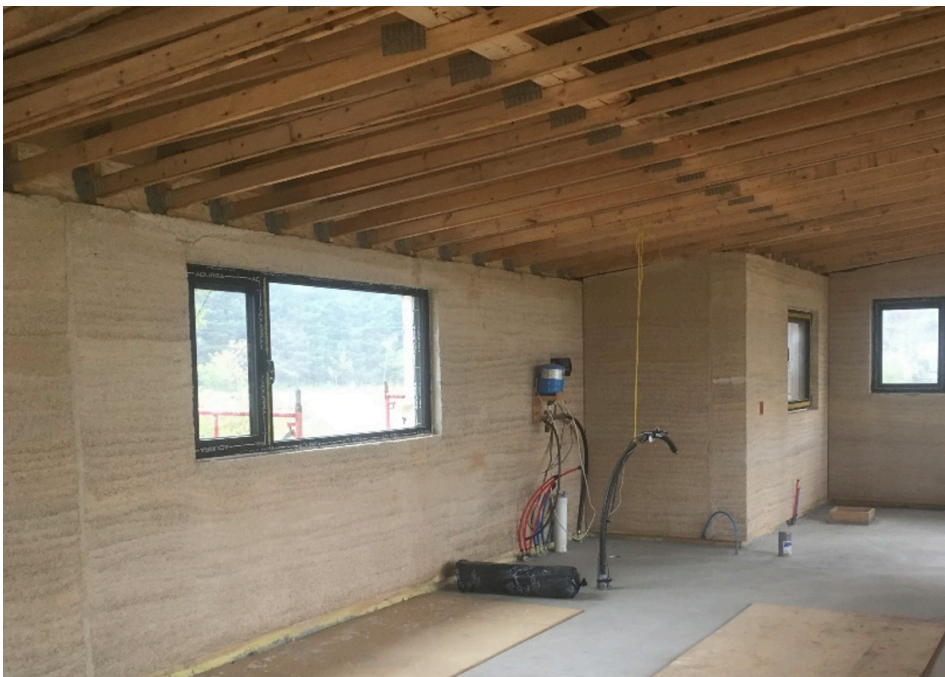
Interior view of walls made of hempcrete
